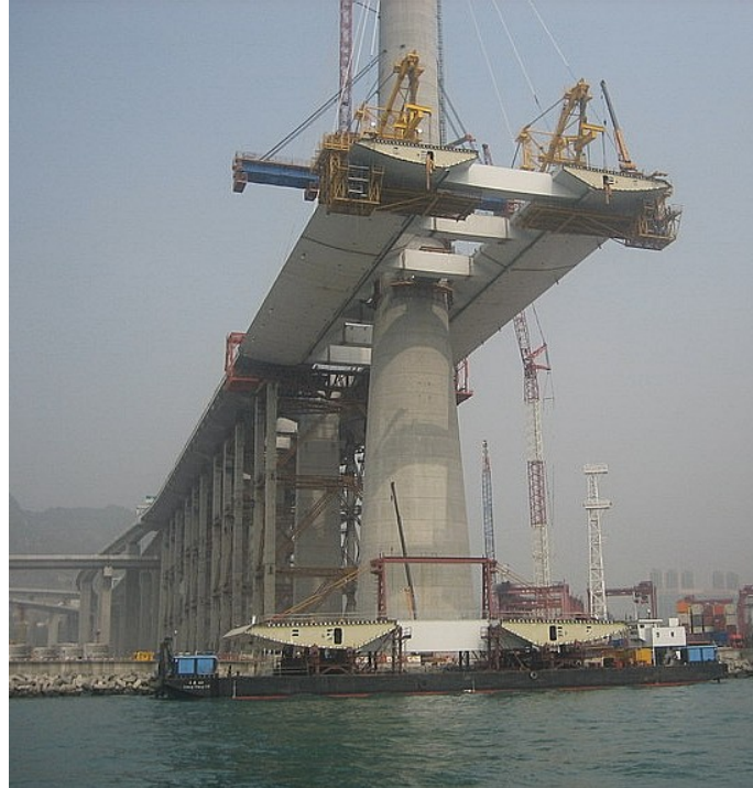
Figure 2 – bridge segment on barge
