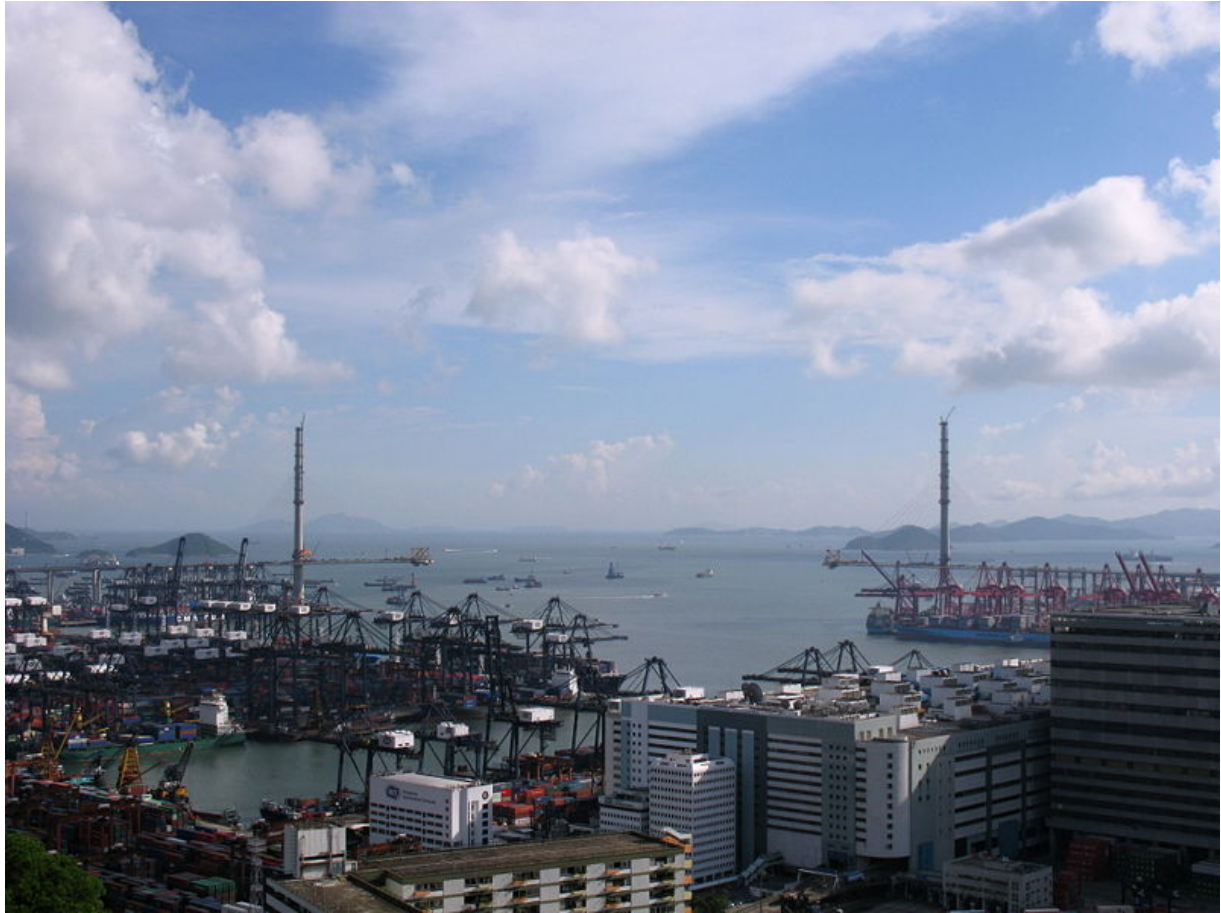
Figure 1 – Stonecutters Bridge under construction
