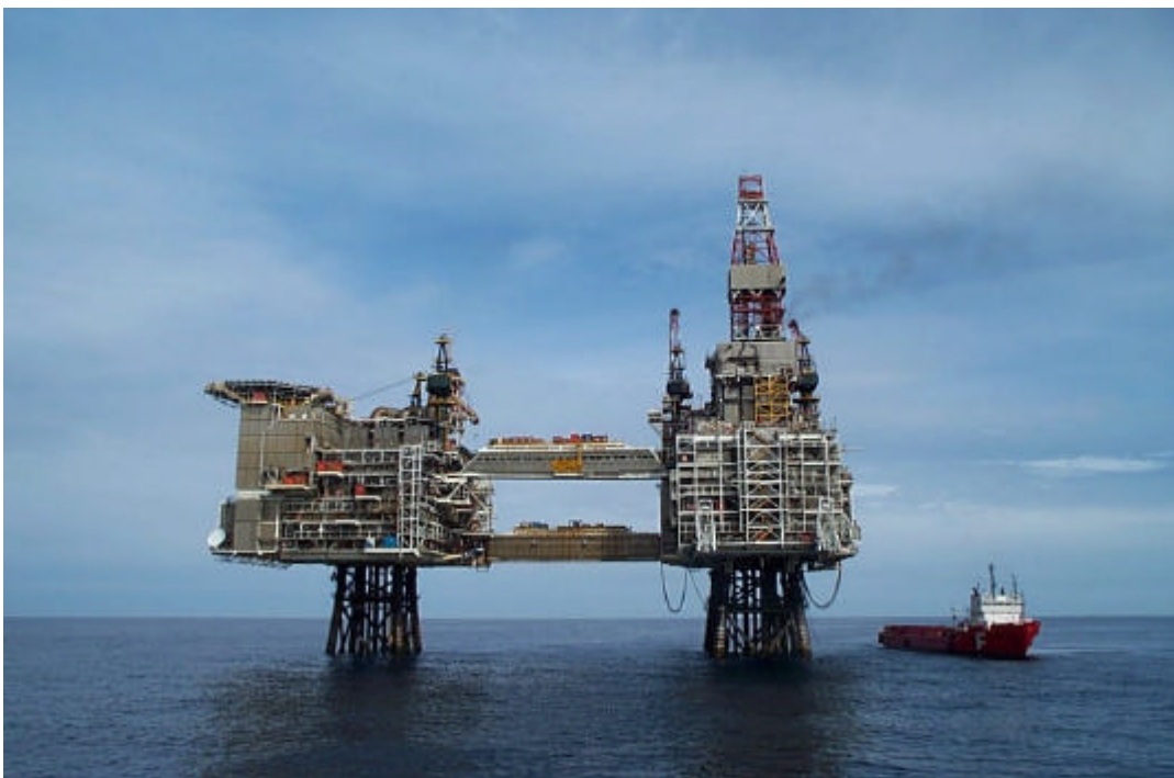
Figure 6, Structure disturbing GPS signals.
