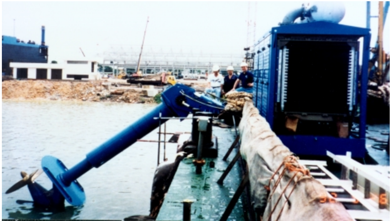
Example 12: Thai cable-lay barge
