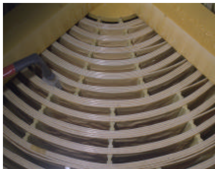
DC Reactor Construction
